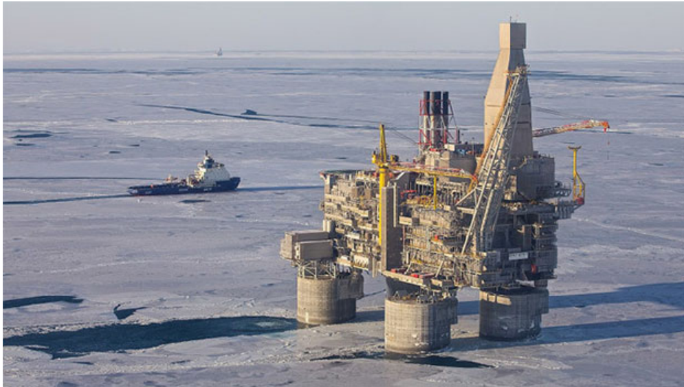
Figure 3-5 An example of a GBS Platform in Arctic Waters, Berkut Oil Production Platform, Sea of Okhotsk, Russia
